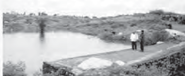
Low Cost Dry Stone Masonry Pond
